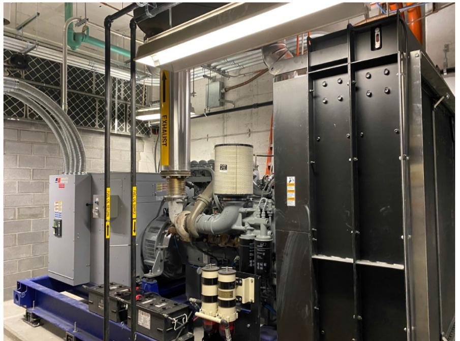
**Figure 1. New 750kW Generator**
