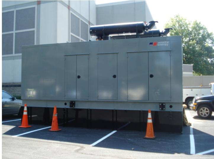
Cynergy provided a design and build project to replace existing paralleling switchgear, replace a 500KW diesel generator and eliminate the need for diesel storage underground and day tanks. The owner came to us with several challenges; to upgrade a under capacity generation system, replace unreliable paralleling switchgear, eliminate the liability of underground diesel storage and diesel day tanks, and provide remote monitoring of the system.
