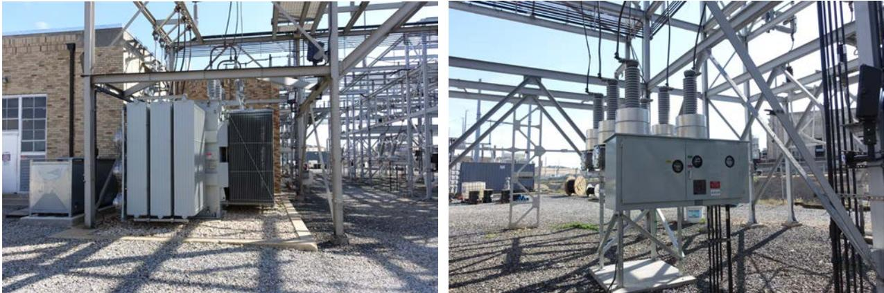
Cynergy performed a \$4,621,543 contract for the DC Water and Sewer Authority at the Blue Plains facility at the existing main electrical substation. The project entailed keeping the existing pumping station operational during the construction process. The new equipment was installed in stages and energized.
