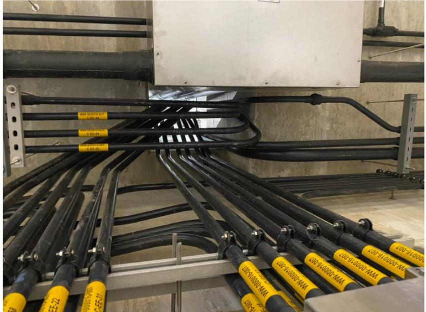
**Figure 2.** Conduits going through floor chase from new EE Pump Room to Electrical Room
